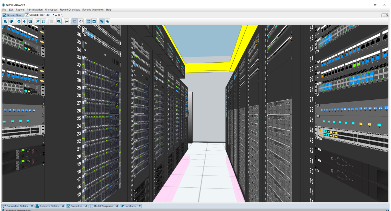
PATCH MANAGER data center 3D overview
